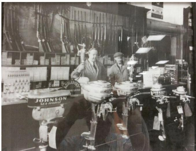
**A 1938 picture of an outfitters store in Alaska with the two most popular outboards in the far north. Johnsons, which were easy to repair and would always get you home and the air cooled Bendix single and twin that would never freeze up and break. No water cooling system to drain.**
