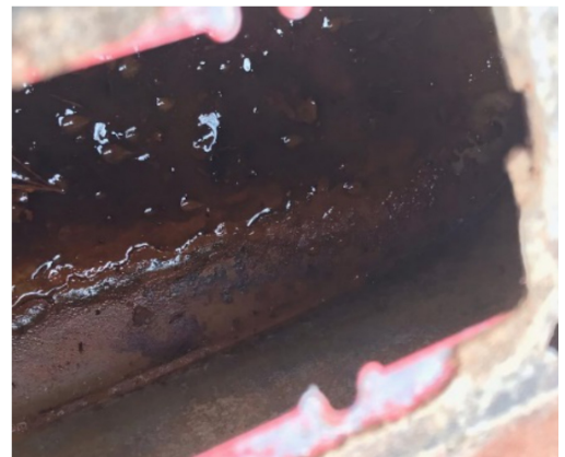
Looking into an old tank for rust.
